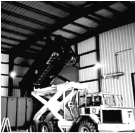
Figure 6.2. Dumping a Roll-Off Container Into a Railcar
